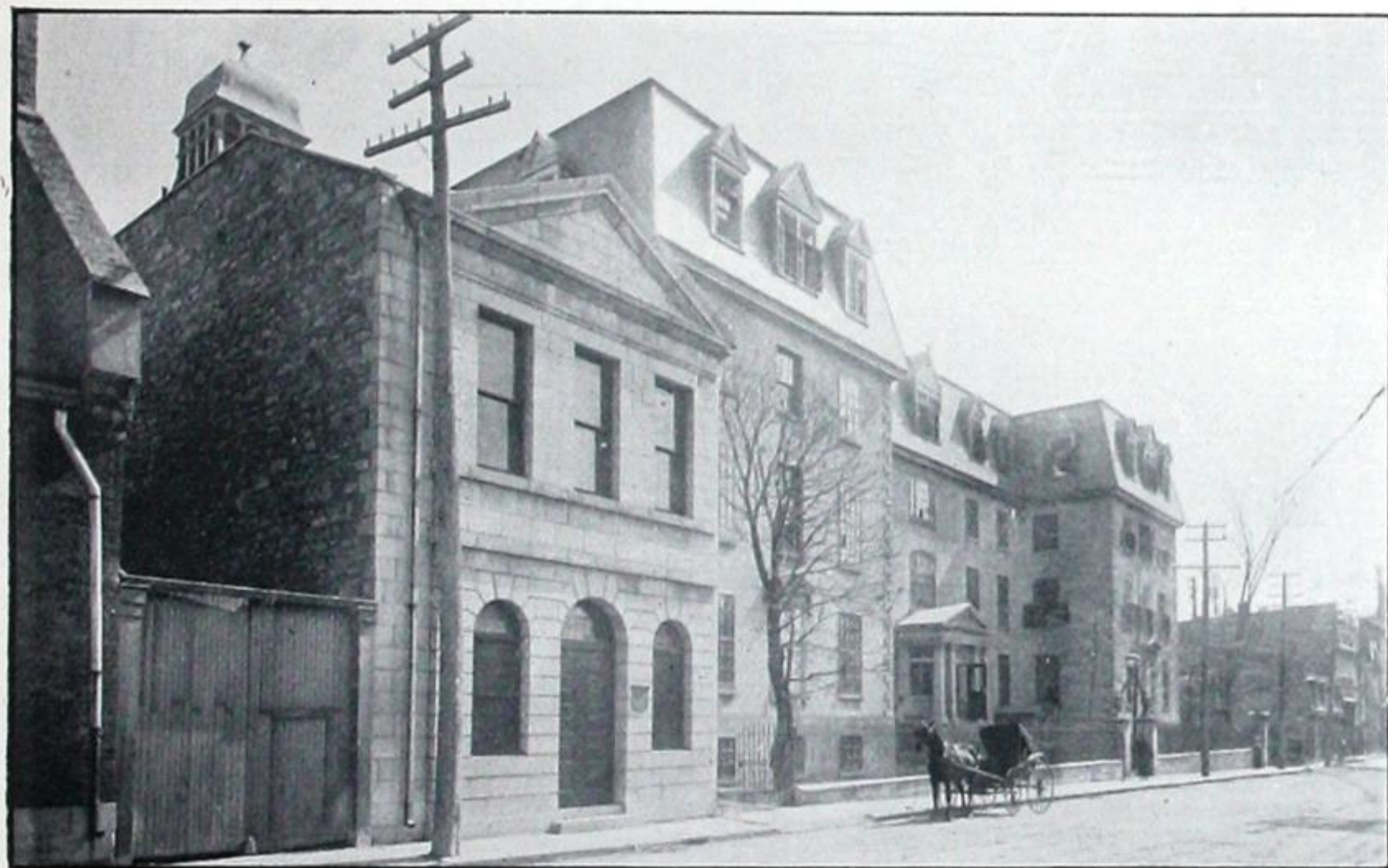
Fig. 187.—General Hospital, Montreal.
